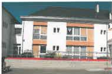
Installation rampe provisoire
